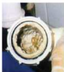
Pipework whilst using pDCB blocks
